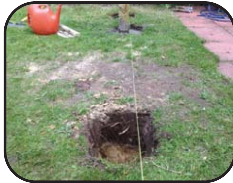
Dig next hole using a string line
