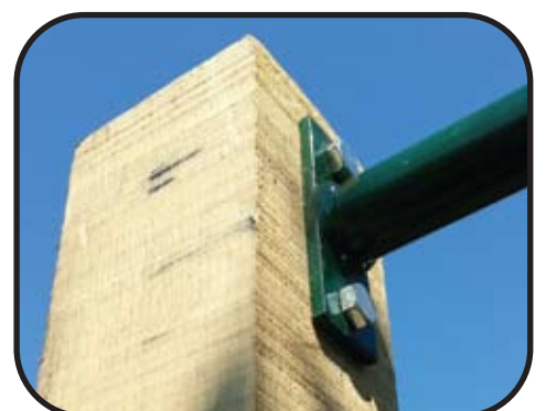
Drill and fix coach washers and coach screws
